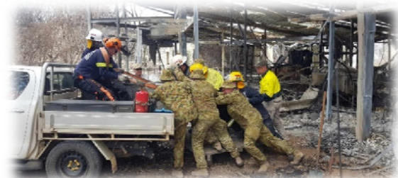
Removing the Fire Arms Safe from Flinders Chase National Park Offices
